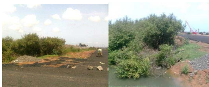
Road construction on Puthuvypu Island
